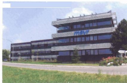
Mayr Headquarters, Germany
